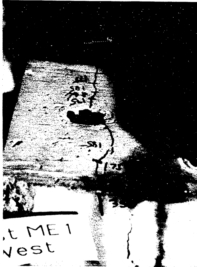
Figure 5.39 Spalling Force Cracking, Specimen ME1
