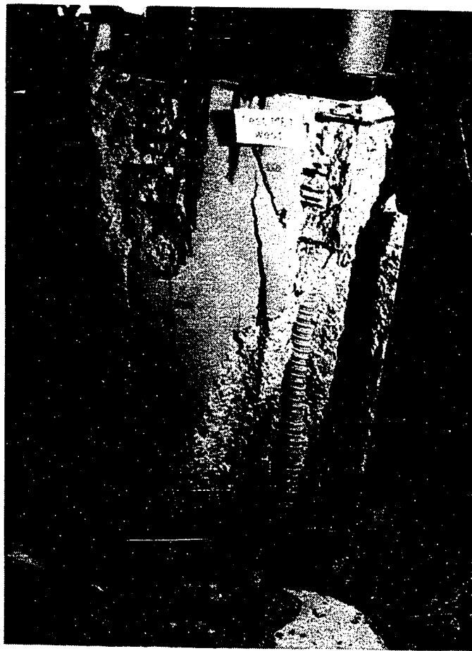
Figure 5.45 Cracking Pattern at Ultimate Load of Test 2, Specimen ME1 (Only Anchorage "B" Loaded)
