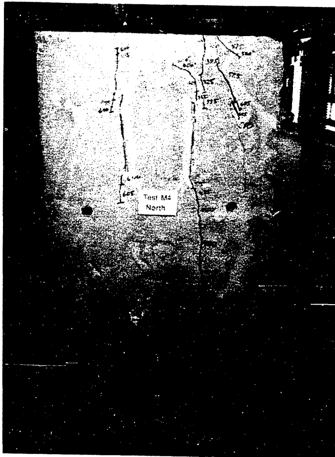
Figure 5.22 Crack Pattern at Conclusion of Test 1, Specimen M4
